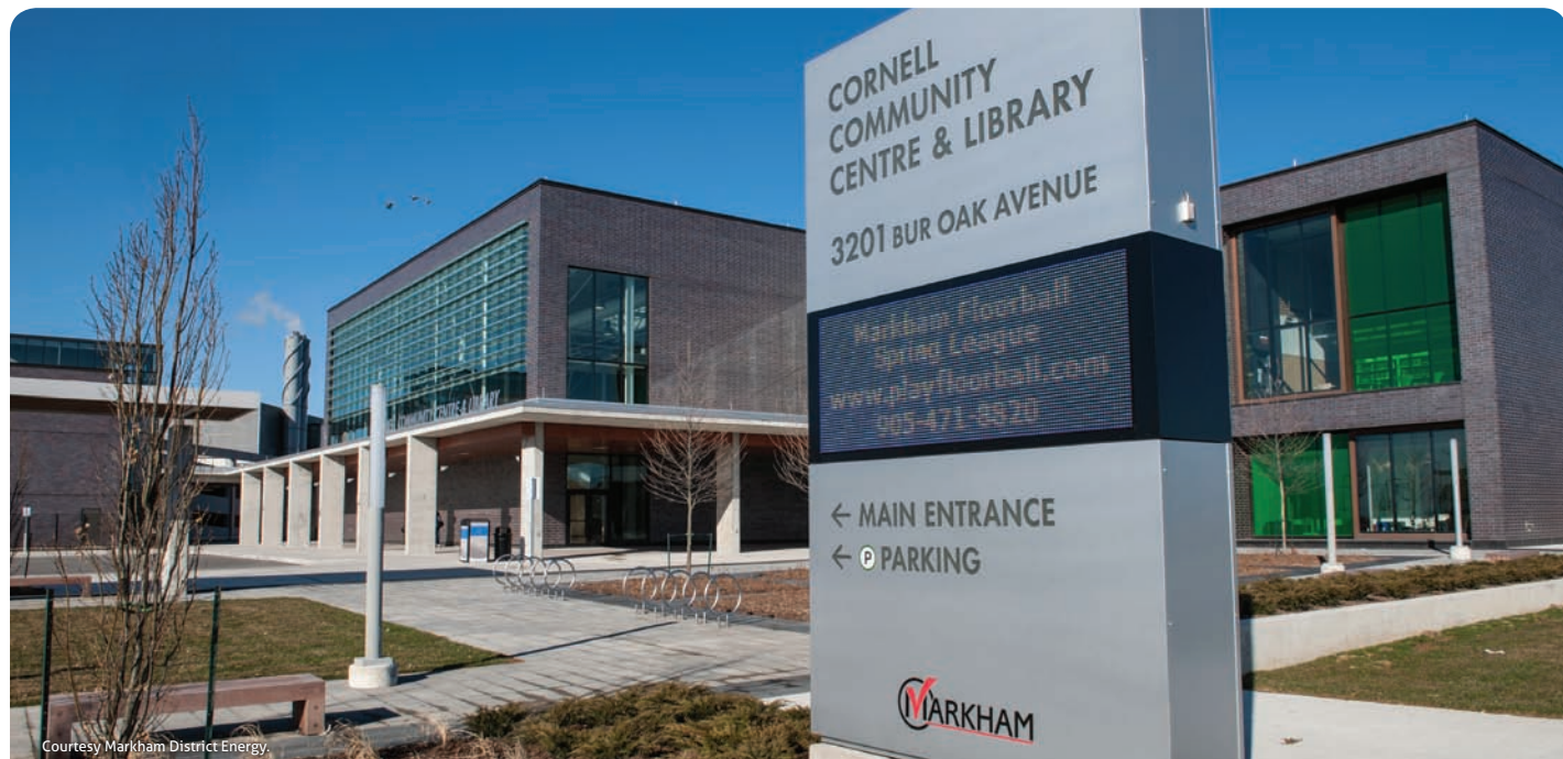
Courtesy Markham District Energy.
