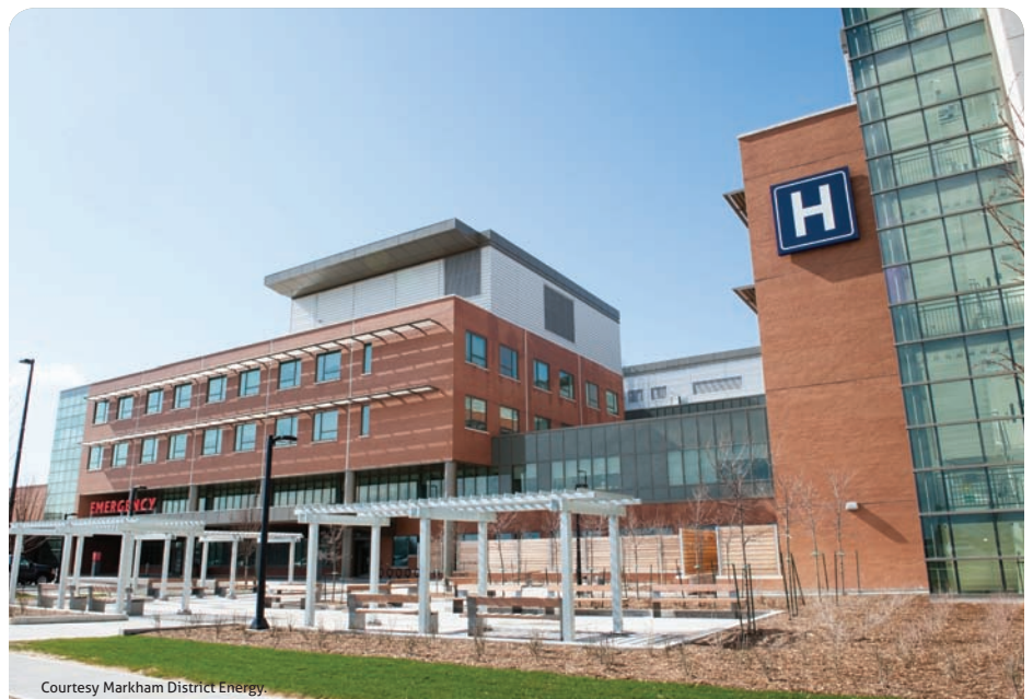
Courtesy Markham District Energy.
