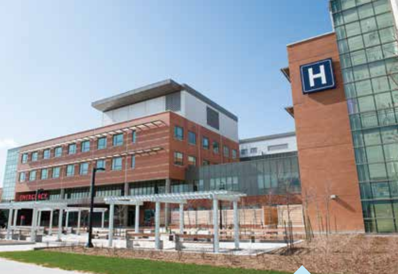
The MDE's Bur Oak Energy Centre services Cornell Centre and provides heating, cooling and power to the Markham Stouffville Hospital
